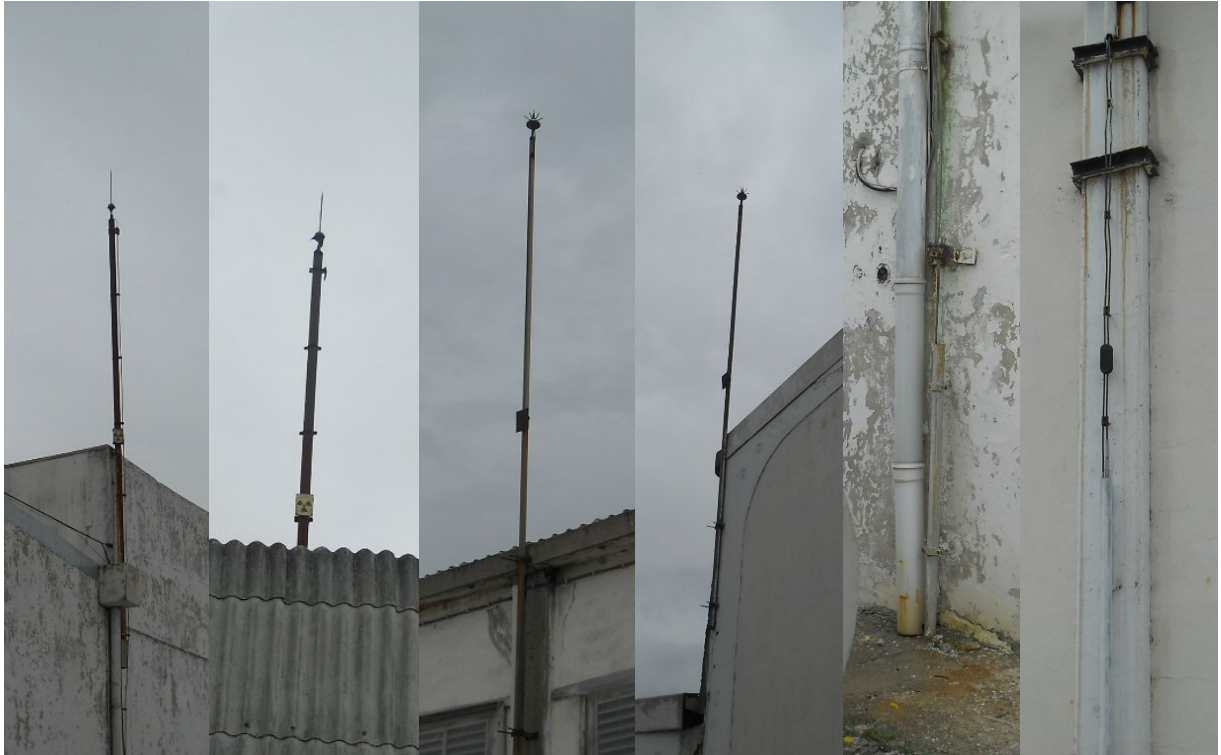
Fig. 3. Samples of radioactive lightning rods and grounding conductors in the factory
