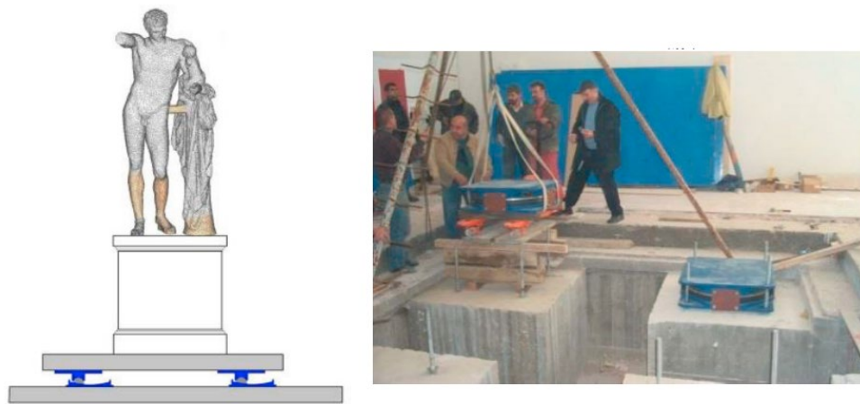
Fig. 2. A seismic isolation application of Statue Hermes is located at the Archaeological Museum of Olympia in Greece [8]
